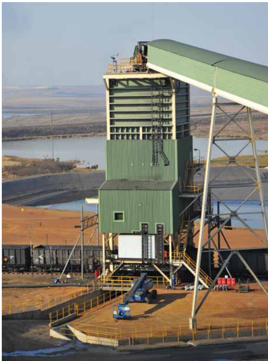
The plant at Goedgevonden complex, Mpumalanga province
