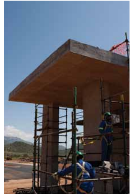
> The mining supplier park under construction
